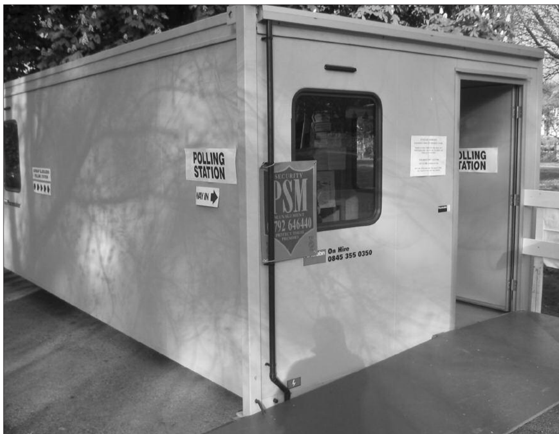
Double whammy: An inappropriate ramp outside a portacabin polling station.
